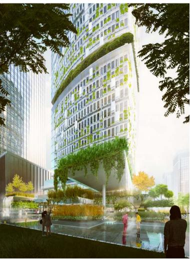
Jian Mu Tower was conceived to occupy the last plot available in Shenzhen's Central Business District, which would complete the skyline of the area's central axis. The 218-meter-high tower dedicates 10,000 square meters of space on its façade to the cultivation of crops. The vertical
