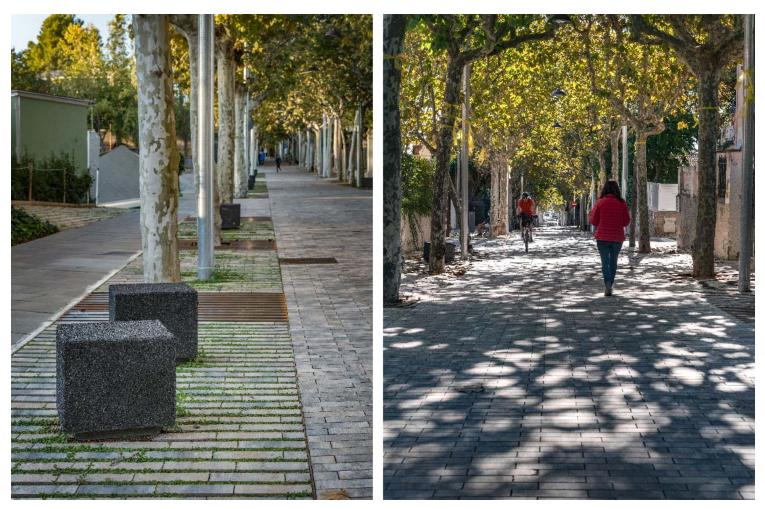
The street is to be paved with 30 x 10 cm precast concrete paving, with different variations in the layout. It will be laid continuously in the central strip, while on the sides, except for the entrances to homes, the joints between the different rows will be widened to enable rainwater drainage and the growth of vegetation. This will provide effective aeration for the tree roots, and avoid the construction of a new network of drains, which has a positive impact on the total cost of the work.
