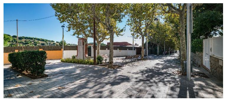
Given the impossibility of walking along the sides of the street, a single platform section is planned, with a single central carriageway where cars and pedestrians can circulate together. This is a central area with two softer strips on the sides that frame the new tree pits, creating new spaces for people to interact, with the possible inclusion of furniture.
