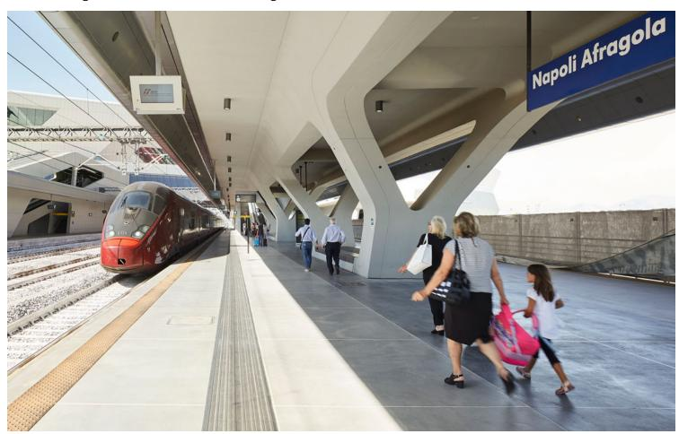
The concrete used within the station is a specific composition that provides optimum performance, with curved structural concrete elements built using technologies initially developed for the construction of the MAXXI Museum in Rome: its wooden formwork replaced by prefabricated steel
