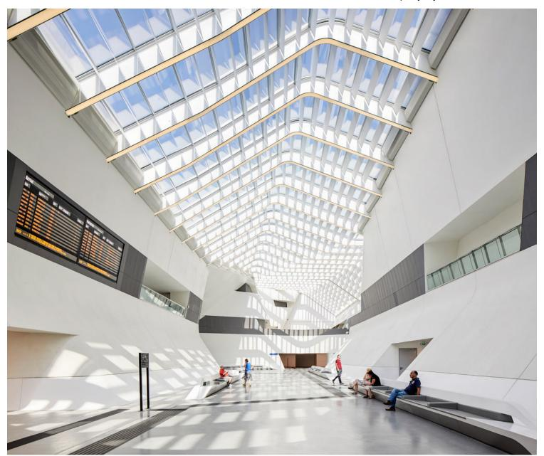
Designed as the extrusion of a trapezoid along a 450m curved path, the elevated concourse is made of 200 differently shaped steel ribs that are clad in Corian®.
