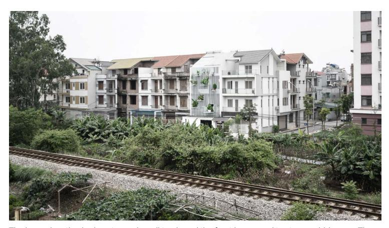
The house location is close to a noisy rail track, and the front is exposed to strong midday sun. Thus, a system of aluminum screen with "balconies" is used for the façade. It creates a new skin that envelops the entire exterior surface, while it still has some openings to bring nature into the house. The "green balconies" use the trees, mostly taking from the green area in front of the house.
