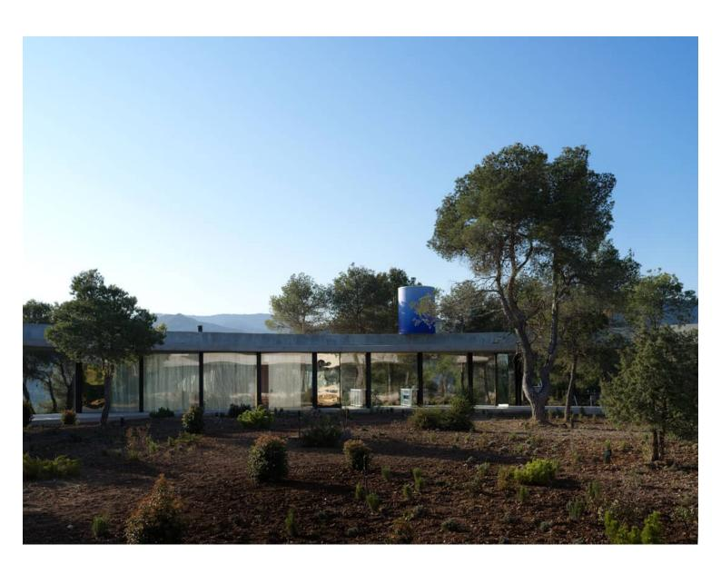
Three of the four are enclosed by glazing set within the steel frames and sliding arcs of curved polycarbonate panels covered with stretched aluminium mesh. All appliances are mounted directly on the columns. The fourth segment serves as a pool house, the floor of which retains the water of the sloping basin within the inner courtyard.
