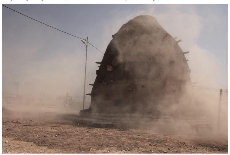
Due to the limited choice of building methods and materials, and the harsh environment characterized by hot summers and cold winters, the beehive style is a viable solution for a school construction. A kind of building technique that does not require high-tensile-strength reinforcements, and can be built quickly with unskilled labour, performing better than tents, cement
