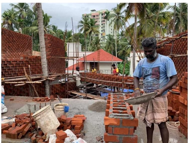
The highlight of the house is a series of sinusoidal slanting walls, gradually moving left and right only to converge at the top for the ferro-cement shells to rest on them. Each wall was specially crafted
