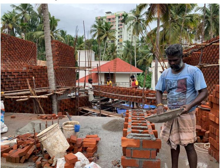
The highlight of the house is a series of sinusoidal slanting walls, gradually moving left and right only to converge at the top for the ferro-cement shells to rest on them. Each wall was specially crafted
