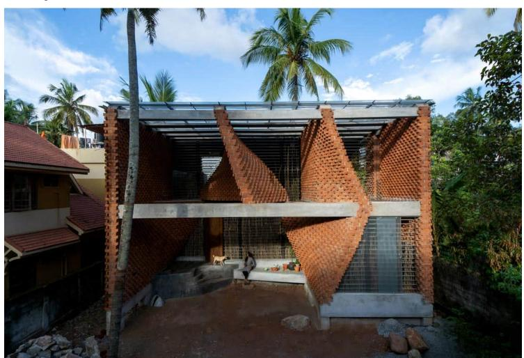
Leftovers from previous stages of construction were used to finish and add character to the space. From scaffolding pipes being transformed into the central staircase and the grills, or the reclaimed wooden planks becoming part of the living room flooring, the idea was to discard nothing as 'waste'. The locally sourced and treated cane was used to add textured screening to the grillwork and furniture, providing vibrance and warmth to the spaces.
