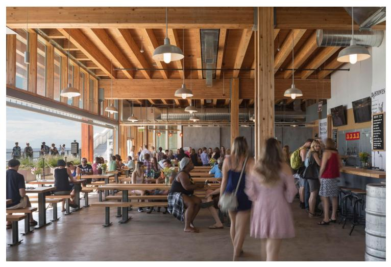
Pike Place MarketFront has a strong Pacific Northwest toughness, employing cast-in-place concrete in combination with engineered timber for the project's base, capped by an open-air structural steel framed pavilion. Railings, canopies and lighting fixtures are in galvanized steel. Large expanses of glazing utilize aluminum curtain wall with glue-laminated mullions to resist heavy wind loads and underscore the industrial feel.
