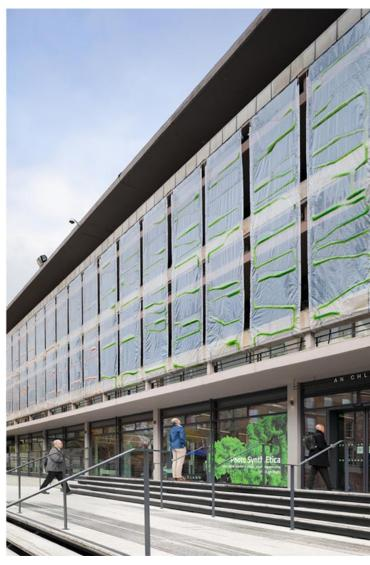
Unfiltered urban air is introduced at the bottom of the Photo.Synth.Etica façade and as air bubbles naturally rise through the watery medium within the bioplastic photobioreactors, they come into contact with voracious microbes. CO<sub>2</sub> molecules and air pollutants are captured and stored by the algae and grow into biomass. This can be harvested and employed in the production of bioplastic raw material, which constitutes the main building material of the photobioreactors. To culminate the
