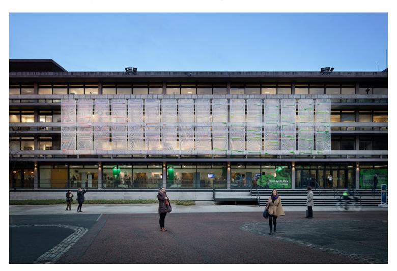
Composed of 16 2x7metre modules, the unique curtain prototype envelopes the first and second floors of the main façade of the Printworks building at Dublin Castle. Each module functions as a
