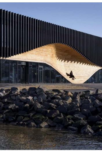
The floating structure and use of glass gives the Klimatorium a distinct contemporary look. The building has two levels and, in terms of scale, it has been adapted to fit in with the existing buildings in the port area. The first floor is surrounded by black-stained wooden slats, which give the building a simple and rustic look and protect it against direct sunlight.
