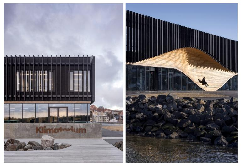
The floating structure and use of glass gives the Klimatorium a distinct contemporary look. The building has two levels and, in terms of scale, it has been adapted to fit in with the existing buildings in the port area. The first floor is surrounded by black-stained wooden slats, which give the building a simple and rustic look and protect it against direct sunlight.
