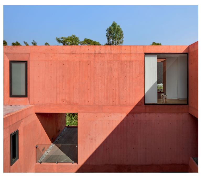
The use of red pigmented concrete as a structural systems and for the finishes makes it possible to generate pergolas, slabs, beams and homogeneous walls, which emphasizes the integrated nature of the project.
