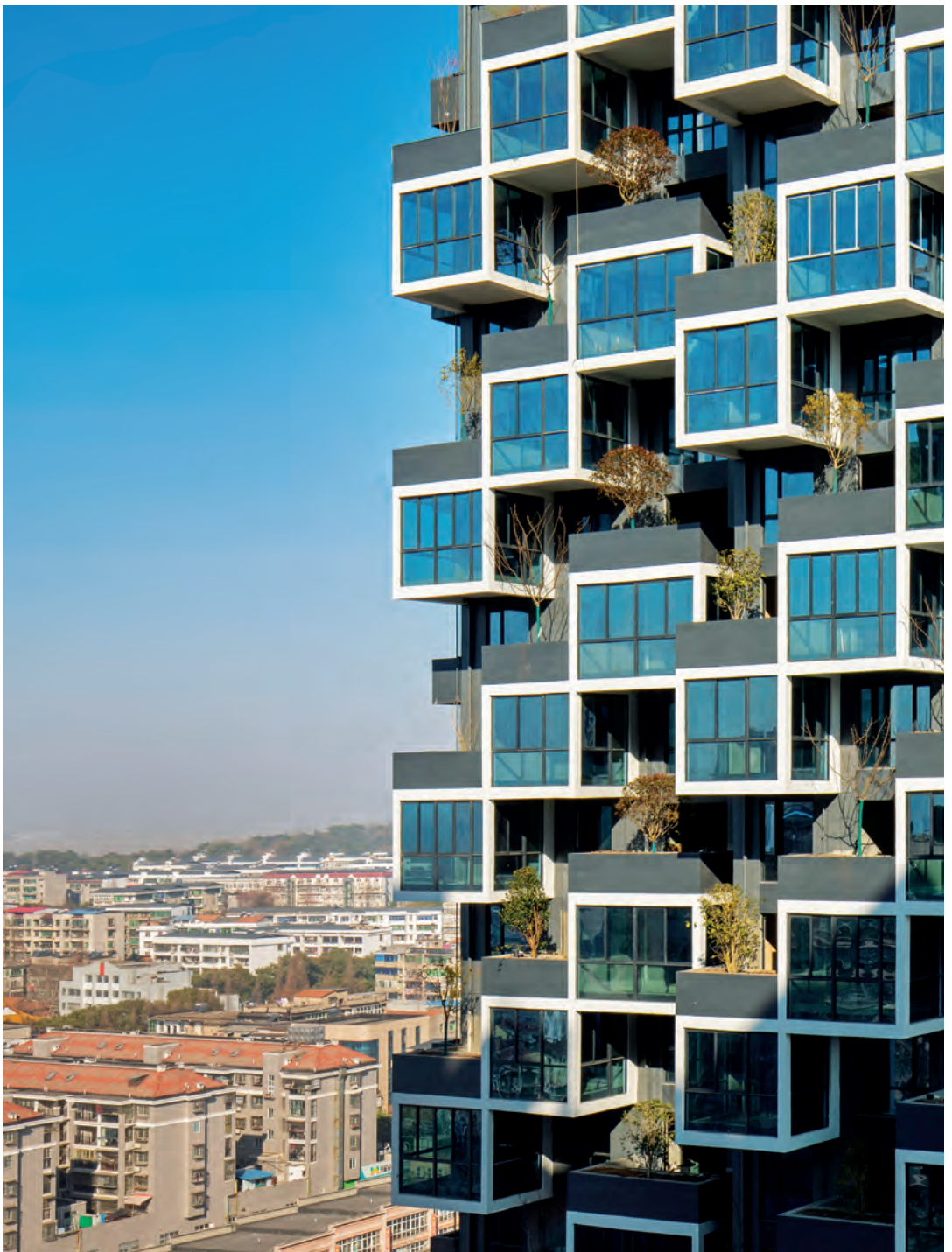
A view of the tree nursery of Nanjing Vertical Forest , Nanjing, China. Stefano Boeri Architetti China, 2021. Photo Credit: Rawvision studio
