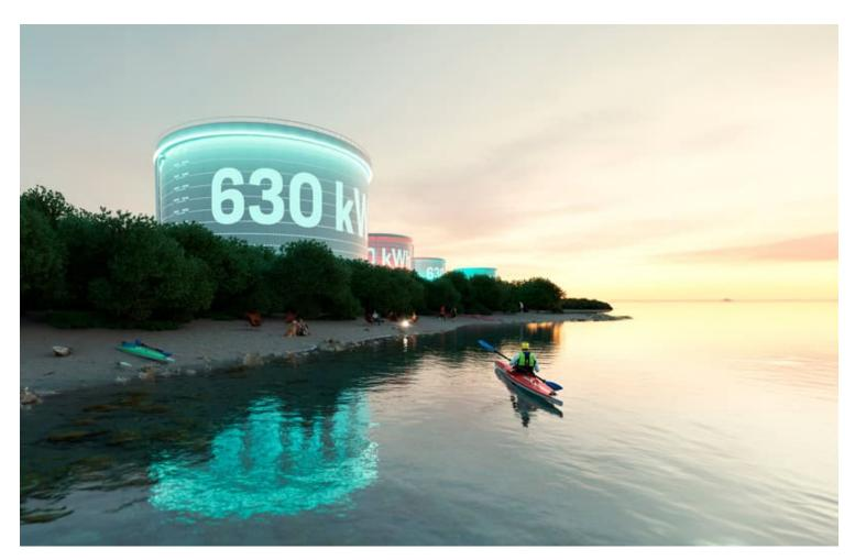
When there is the need to store power, seawater is pumped up into the tanks and turned into potential energy. Conversely, when power is needed, the stored seawater is used to produce hydroelectric energy, pouring water back into the sea. The system functions as a small "pumped hydroelectric" plant. The solution is fully renewable as the energy needed to pump up seawater is provided by agrivoltaics – elevated photovoltaic panels scattered across a publicly accessible urban park.
