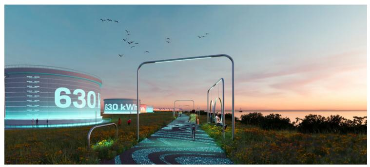
Suggesting new ways to reuse former industrial facilities, the design employs renewable energy sources in an integrated way. At the core of the project are six former oil reservoirs – each of them at a height of 15 meters, totaling 110,000 cubic meters of capacity – that will be turned into water batteries.
