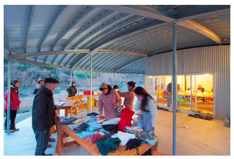
Therefore HOME-FOR-ALL decided to build a space for residents to be able to meet easily in the centre of the island; a big roof, with space for everyone underneath it. The design is a circular main framework made of steel, with a light rounded roof sitting on top. Below the roof there is a semi-outdoor terrace and a living room. The living room can also be opened up to become one with the terrace.
