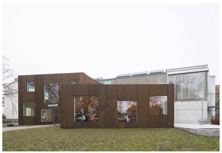
The corten steel, favored by sculptors ever since the material was invented, handles the adjacent historic red brick architecture as well as the rough materiality of the existing concrete volume, yet contrasts to these with the potential of sharp detailing inherent in a panel material. The free
