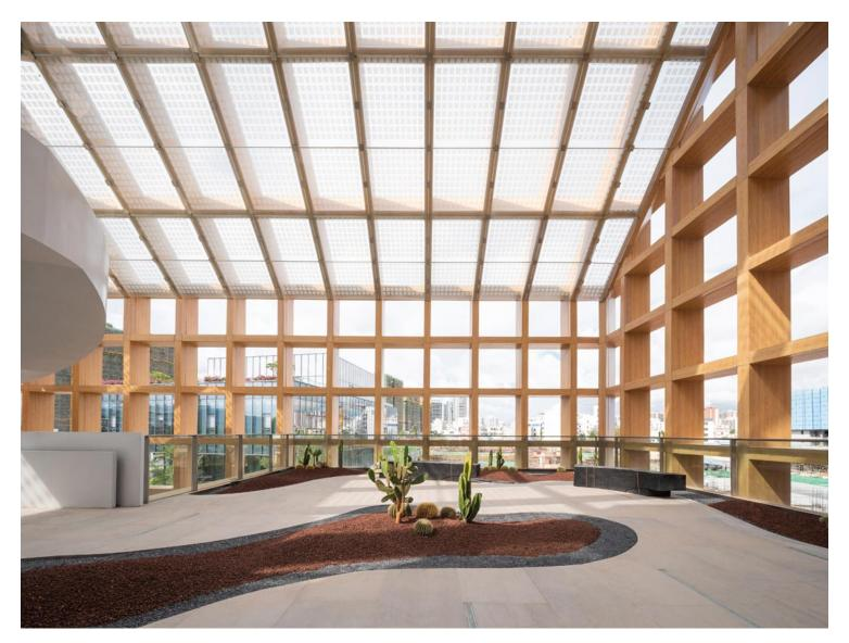
In the interiors, glare-free natural light filters below the horizontal ledges into offices and research zones. Sunlight permeates the partial translucent roof over the outdoor areas, while open façades ensure optimum natural ventilation. Public half-climate spaces alternate with air-conditioned zones on all levels as required by the program. On the ground floor, a continuous perimeter overhang provides sheltered access and open-air circulation.
