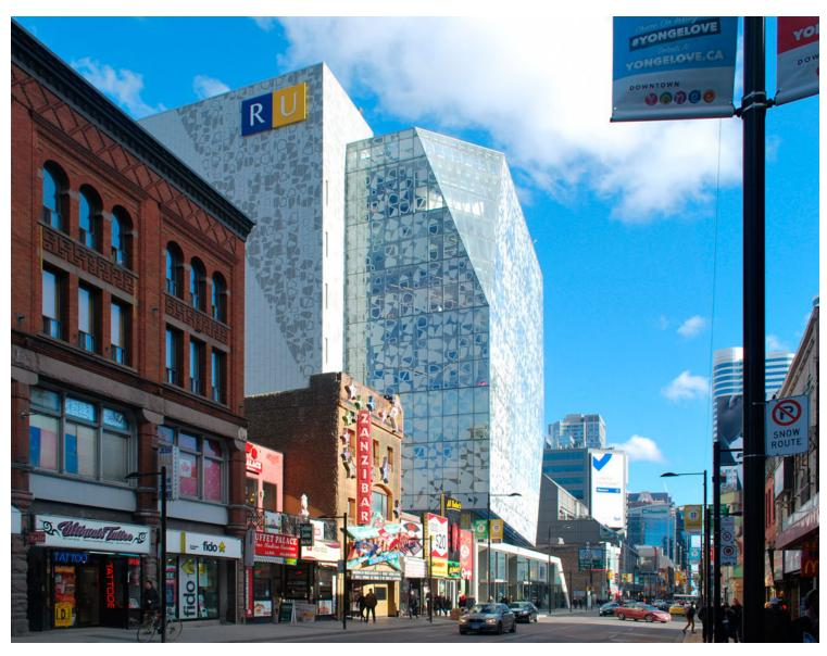
Functioning like cloud cover, the frit modulates the light quality to range from 'overcast' to 'partly cloudy' to 'sunny' to further diversify the interior conditions and allow students to have a different experience every time they visit the building.
