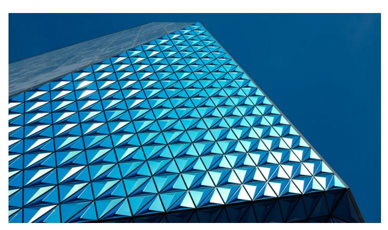
The facades of the building are composed of a digitally-printed fritted glass that envelops the rugged armature and pared-down aesthetic of the exposed concrete structure. The varying façade pattern controls heat gain into the building and frames views of the city grid and nearby buildings from the interior, acting as a traditional framed window without actual frame constructions.
