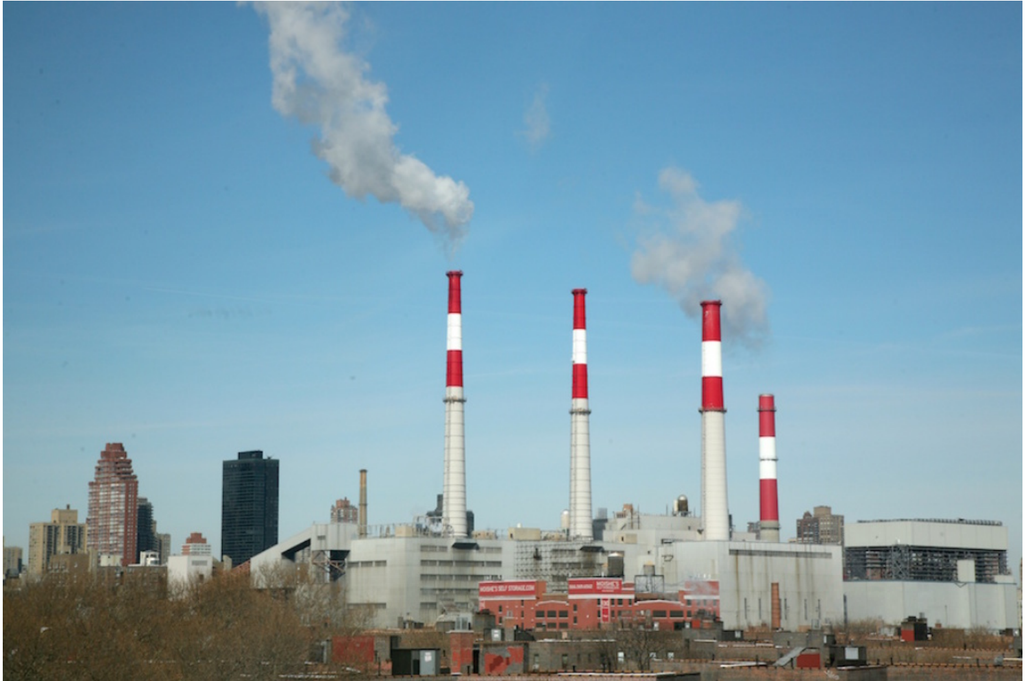
ConEdison's electric power generating plant in Queens. (Flickr/Vincent Desjardins)
