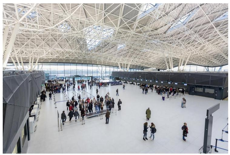
The flexibility of the conceptual scheme allows for adaptability with the open spaces, formed largely by a 14.4 x 14.4 m modular column grid at the concrete base. A post-stressed reinforced concrete structure is built on a grid pattern with various spans that are multipliers of the base module: 7.20 m, 14.40 m etc.
