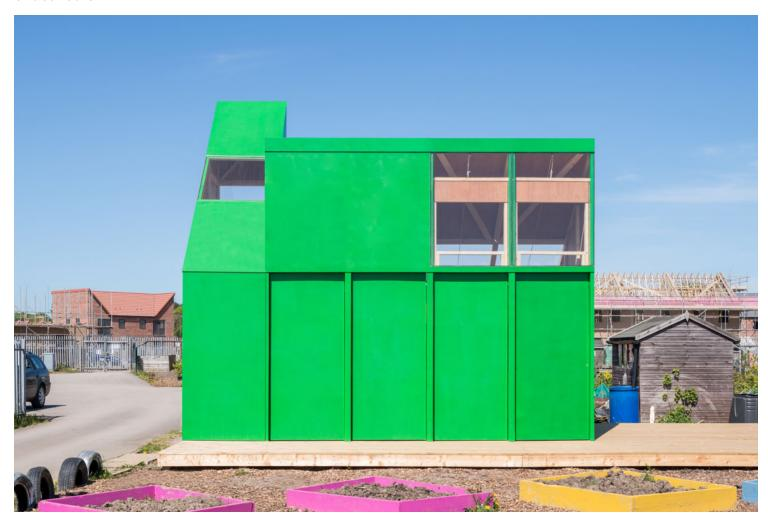
The structure is a lightweight timber frame supported on a suspended deck that sits on ground-penetrating metal foundations. The southern wall is designed with large, pivoting, counter-weighted doors that lock down securely at night and in winter and open up to the allotment to provide an extended canopy with a deck
