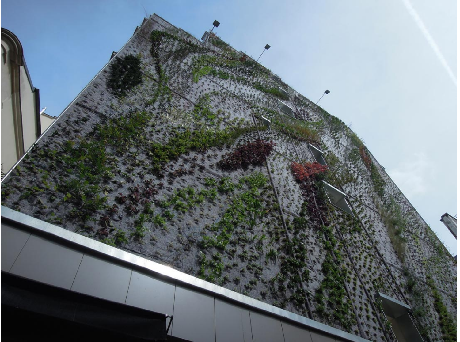
The green wall at its very beginning, April 2013
