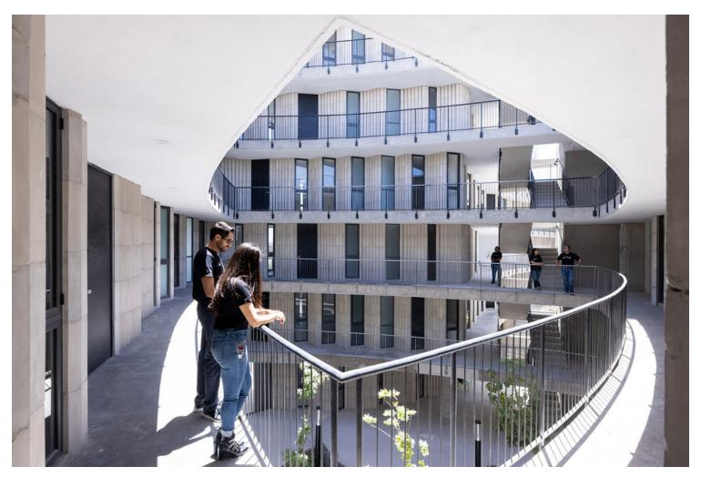
Our project creates 60 condo units as a vertical housing block at the city's center. The design maximizes the plot's buildable footprint and generates two interior courtyards that provide cross ventilation to each unit, with parking and a commercial ground floor.
