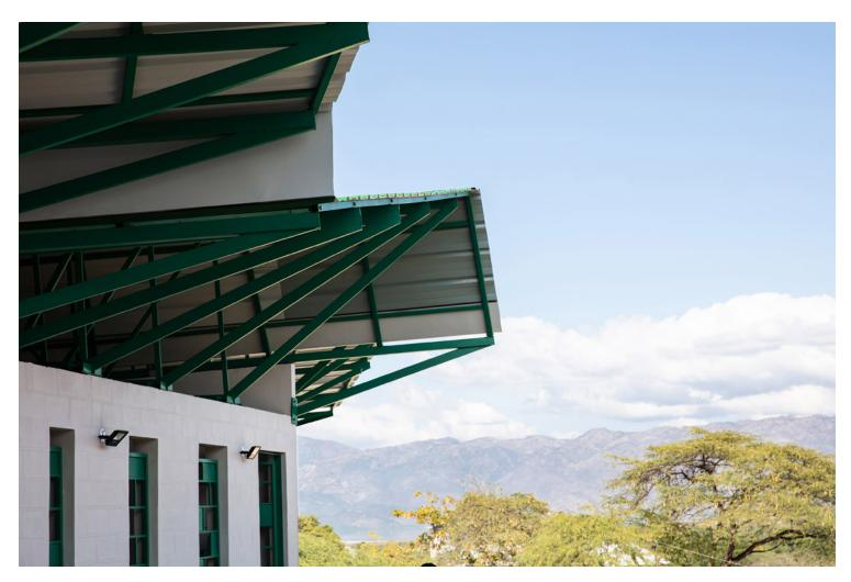
The building emerged from carefully studying and combining the only affordable materials – CMU block, concrete, and corrugated steel roofing – in order to increase air-flow, provide natural light and security, and control sound transmission between classrooms. The façade's rhythm of reinforced piers and openings, which is a big part of the school's identity, is based on playfully shifting the CMU block piers which transfer the bearing, up-lift, and shear loads down to the foundations.
