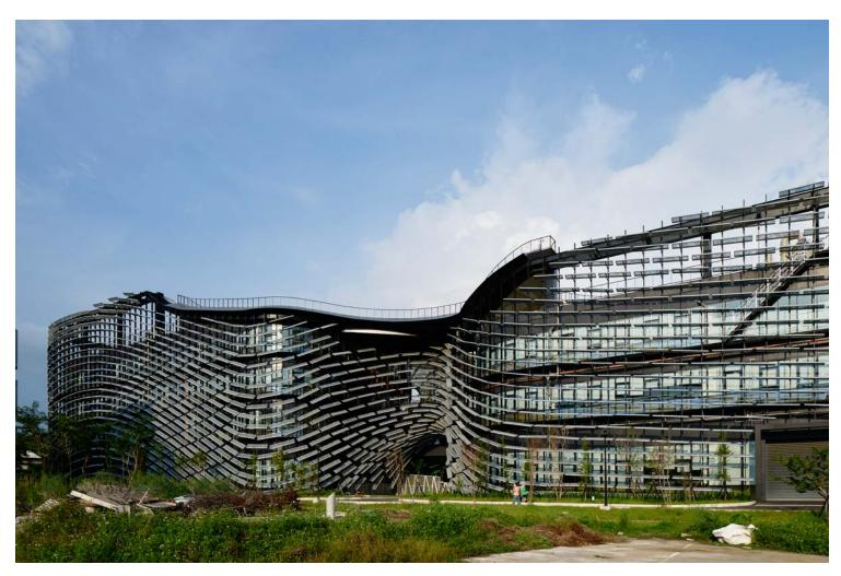
The fins resemble a school of fish- the fins are positioned at various angles, while as a whole creating a large flow and giving a dynamic impression to the building.
