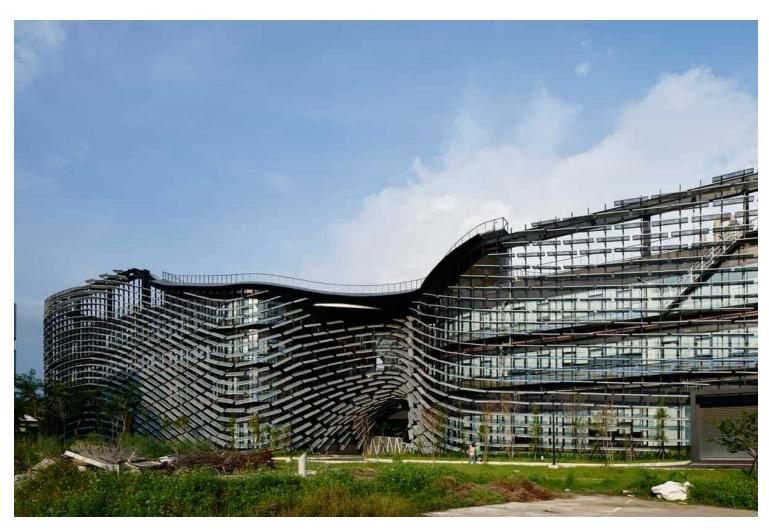
The fins resemble a school of fish- the fins are positioned at various angles, while as a whole creating a large flow and giving a dynamic impression to the building.
