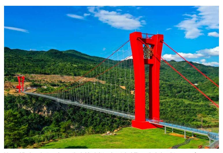
Meanwhile, in order to enhance the bridge's lateral sustainability and wind-resistance performance, the designers adopted an oblique wind-resistant cable system, which is fixed to concrete anchors. Moreover, considering the adverse influences of karstification and special residual silty clay on the site, they worked to ensure the safety performance of the bridge during the design and construction phases.
