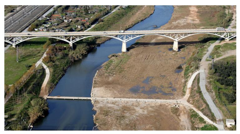
The floodable structure crosses the river at a point where the riverbed is relatively narrow, upstream of where it meets the Torrelles Stream; it provides a crossing for foot and bicycle traffic, as well as for service vehicles, as long as the rising waters don't make it impassable. From the two gravel paths on the banks, the difference in height, of five or six metres, is resolved with concrete ramps that run down into the riverbed.
