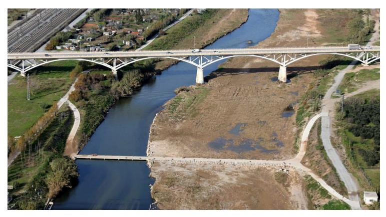
The floodable structure crosses the river at a point where the riverbed is relatively narrow, upstream of where it meets the Torrelles Stream; it provides a crossing for foot and bicycle traffic, as well as for service vehicles, as long as the rising waters don't make it impassable. From the two gravel paths on the banks, the difference in height, of five or six metres, is resolved with concrete ramps that run down into the riverbed.
