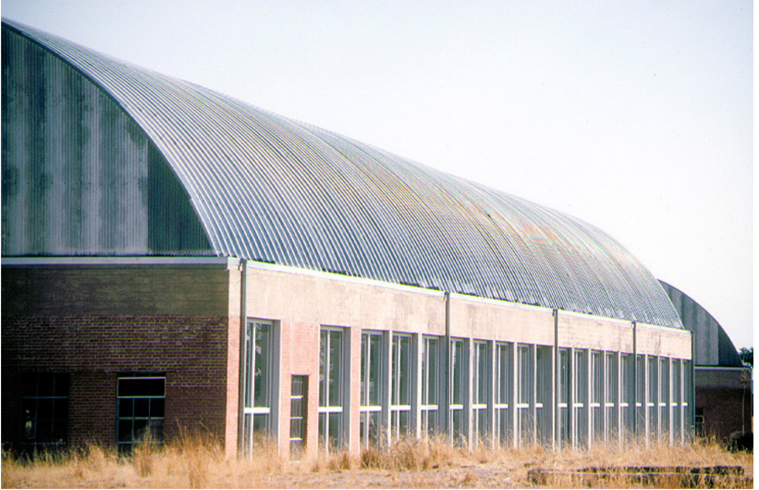
Front façade and side windows. Artillery Sheds. (Gillermo Zuaznabar)
