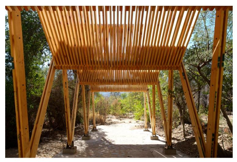
The proposal consists of a structural system that understands the canopy as hut, as shelter for the family. It avoids formalizing the shed as a sum of vertical supports for the horizontal plane and rather seeks continuity between the roof and the support points.
