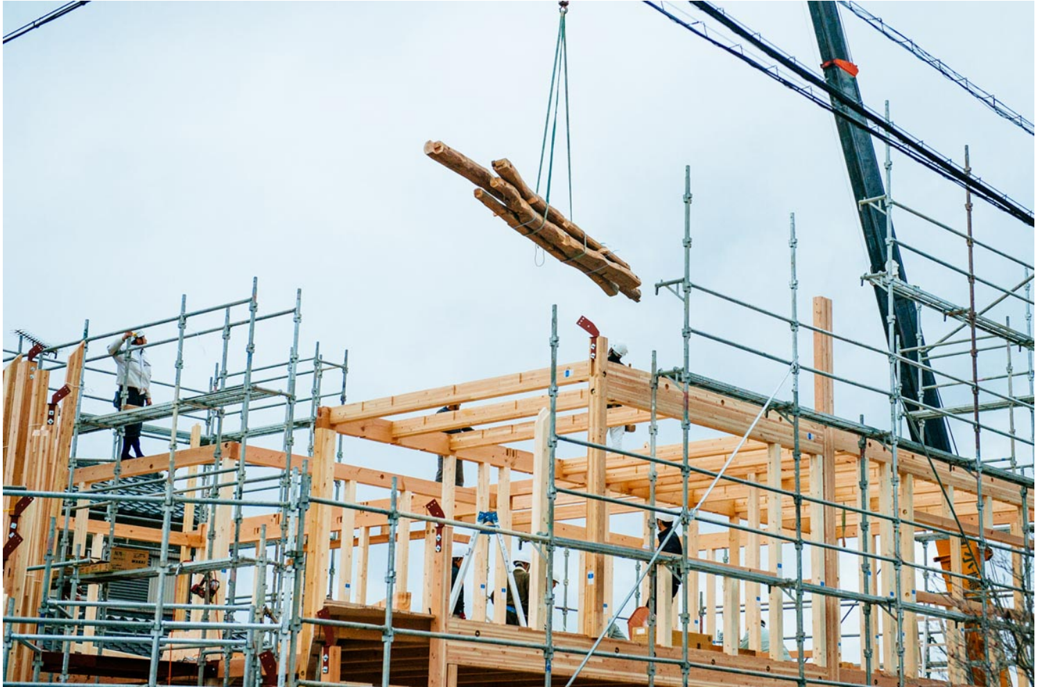
Clover House under Construction
