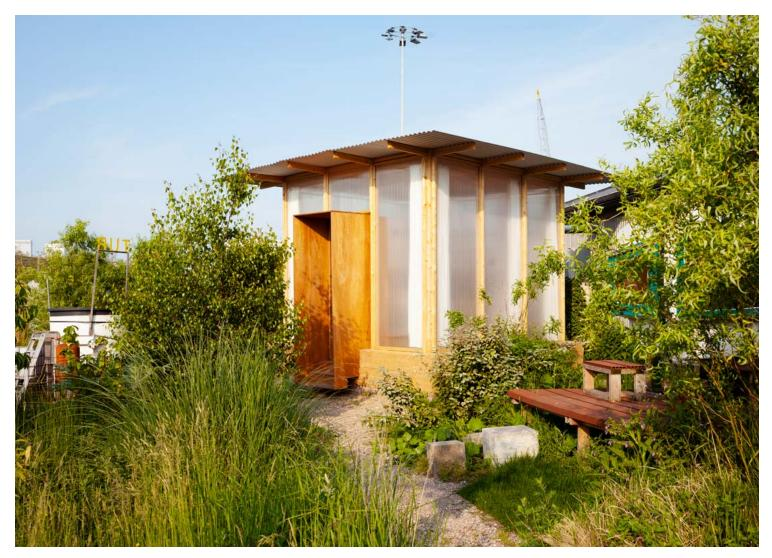
The cabin sits in the heart of a wild garden in Rotterdam; each element and detail is visible from both inside and outside, offering a permanent dialogue with the garden. The door is lifted off the ground and attached to the transparent cube. The rammed earth base is both a wall and a floor, combining two functions, emphasizing its archetypal form. The aluminum roof floats and reveals the timber
