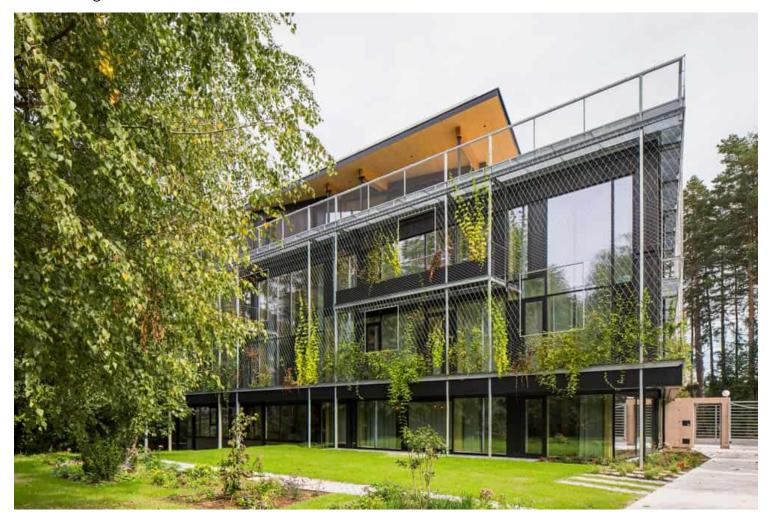
For the façade, a traditional Japanese method of wood preservation, known as yakisugi, was used. Slightly charred and thus carbonized, the façade is both waterproof and durable without the need for further painting, while also protecting against insects. The basement and the building core are made of reinforced concrete. Wood was also used for the mullion-transom-façade, the windows,
