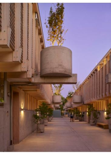
The second floor contains the bedrooms in a space attached on both sides to its neighbors, forming two long rectangular pavilions. The laminated wood structure is arranged under a continuous modulation of 77 cm. with the upright elements exposed to the outside on the second floor. Towards the courtyards, they frame the bedroom windows, preventing the view of the neighboring houses. Towards the walkway, they frame a series of larch tiles, creating a wall.
