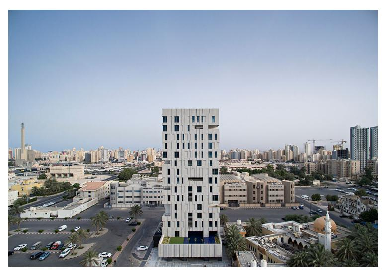
Understanding and reinterpreting local environmental techniques is one of the main targets of this design. The services core of the building is thus located on the southern wing, in order to minimize sun exposure and consequently reduce energy consumption, acting as a thermal barrier to the rest
