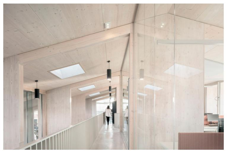
Roof, plates and floors are created from cross-laminated timber. The chief material matches the stored timber shaping the company's precincts.
