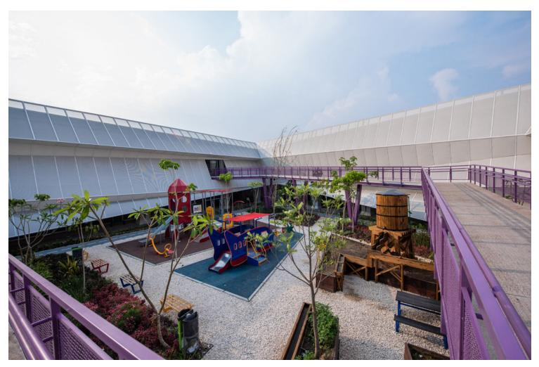
Despite its unique aesthetics, the building reduced costs by making efficient use of national materials such as stone slabs from the region and expanded metal sheets. The use of eco-technologies was an important consideration. Rainwater collection and a double façade, which acts as an element of solar protection and at the same time provides daylight and natural ventilation, reduce energy consumption.
