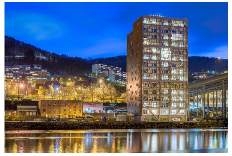
The main principle of the building is independent modular units with their own walls, roofs, ceilings and roof construction, stacked between the main glulam framework. All gaps are closed with insulation, and the building is coated with an outer shell to weather protect all the individual parts and the gaps between them.
