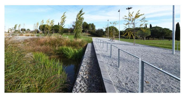
The topography of the land was changed to create a depression by digging out the central part and filling the margins with the same soil; likewise, three platforms were installed across it on rows of prefabricated gabions. Temporary flood areas were created at these interruption points that redirect the surface runoff towards the depression.
