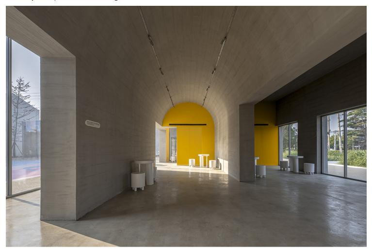
The building adopts a cast-in-place concrete structure. Corresponding to the CPC Community center on the west side, the Qinchang Village Town Hall also plays with the geometry and motif of arches, a typical component in the local traditional semi-underground dwellings. Based on the geometric prototype and modules previously set up on the west side, arches were further abstracted and evolved from planar models into vaults, catering to various spatial and programmatic
