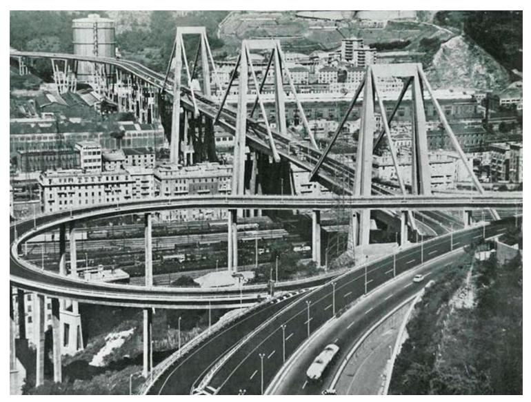
Built between 1963 and 1967 by the Italian company Condotte d'Acqua, the bridge had a length of 1.18 kilometers, a height of 45 meters and three large A-shaped concrete supports that reached 90 meters. The length of the main span was 210 meters.
