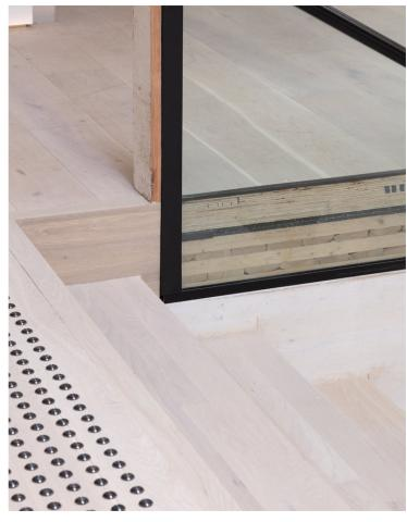
"Because of the type of movement – dance, performance – happening in that space, it was important for the system to be a proper sprung-wood floor. The clients wanted the warmth of real wood but also wanted to avoid replacing it in the case of a big flood event," explains Mandl.
