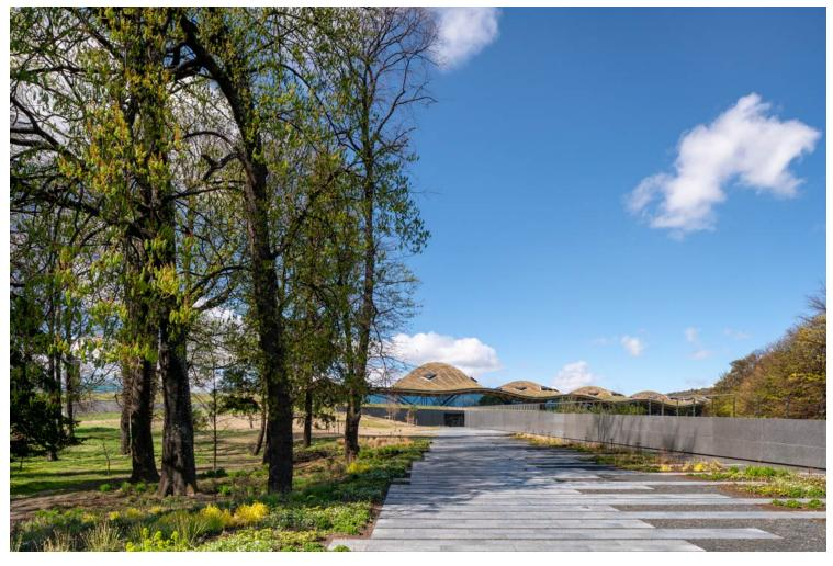
The new distillery will enable production of The Macallan to increase by a third if required. Internally, a series of production cells are arranged in a linear format with an open-plan layout revealing all stages of the production process at once. These cells are reflected above the building in the form of a gently undulating timber roof. Grass-covered peaks rise and fall from The Macallan estate grounds, signaling to approaching visitors the activities housed beneath.
