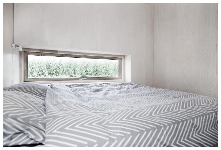
The inside is entirely clad with birch plywood while the external finish is made of vertical untreated larch panels which will turn to a lighter silver tone over time, allowing the house to adapt to its surroundings.
