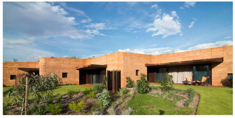
The rammed earth wall (construction) is composed of the iron rich, sandy clay that is a dominant feature of the site, gravel obtained from the adjacent river and (bonded with) water from the local bore (hole).
