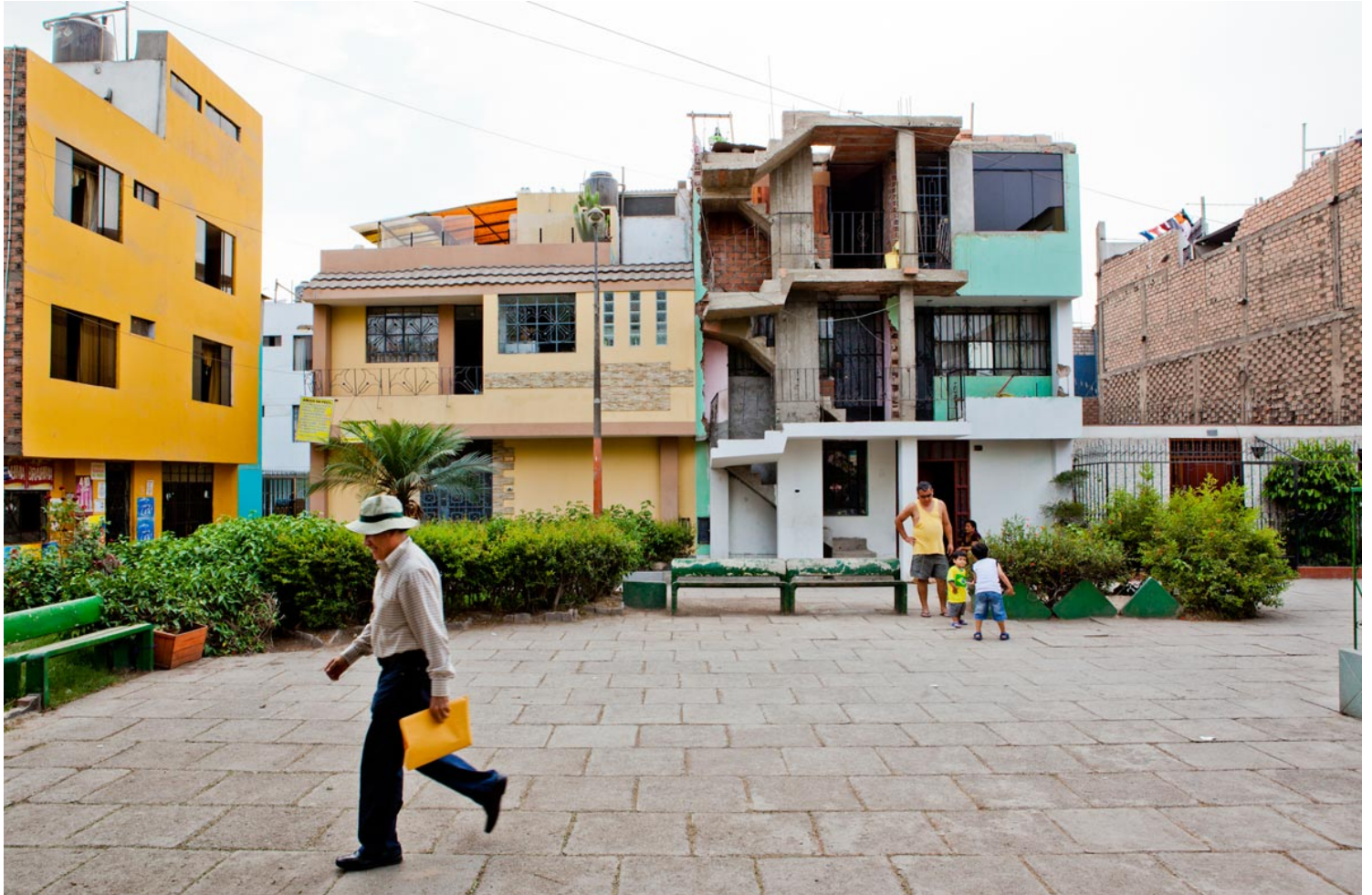
A courtyard and one of the inhabitant-modified houses in the experimental Proyecto Experimental de Vivienda (PREVI) project near Lima, Peru, 2011
