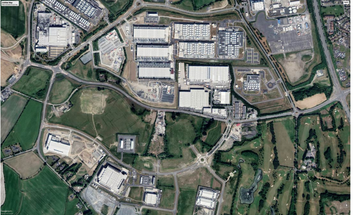
Fig. 4. Aerial view of Google and Microsoft data centres, Grangeacastle Business Park, Co. Dublin.
