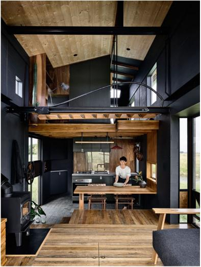
The staircase at the kitchen bench can be moved out of the way by turning the wheel by the entrance. This turning mechanism engages with the house frame during transport but operates the
