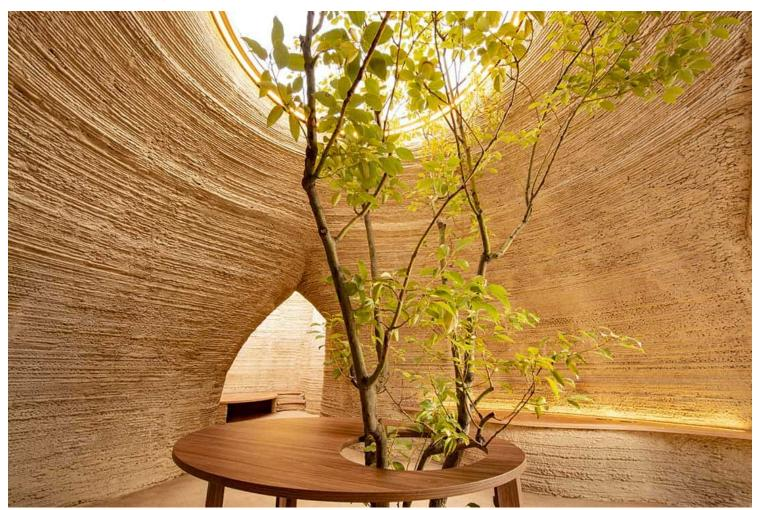
The technological research of WASP, specialized in Kmo 3D printing from raw earth, has led to an innovative 3D printing technology called Crane WASP, the first in the world to be modular and
