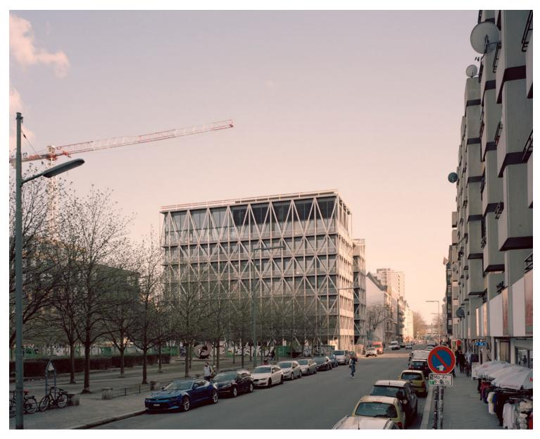
The structural system of the new house is designed as a network with minimum materials used to achieve the maximum load capacity. All the elements perform the same function and only achieve stability together. It is a system without hierarchy. The architectural appearance of the new house for the *taz* reads as a structure and as a symbol of the organization at the same time.
