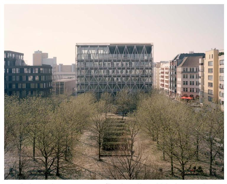
Externally, the network structure appears as a filigree layer with French balconies. It spans the new building and gives it its lightness. The 13-meter-deep office areas create a workshop atmosphere and allow for a variety of ways of working. In the center of the building, a vertical staircase sculpture connects the floors.
