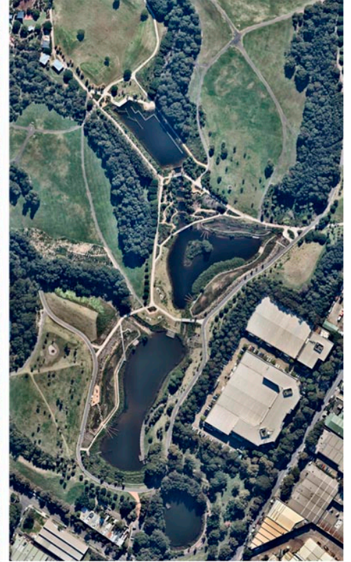
After Construction May 2016
