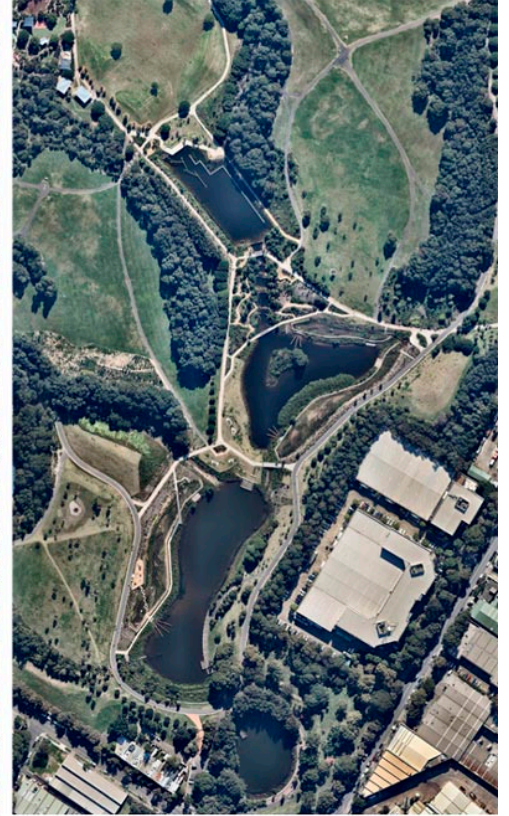
After Construction May 2016
