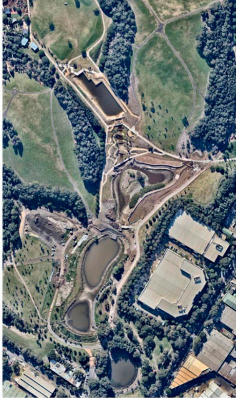
During Construction June 2014
