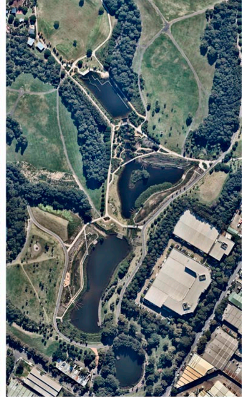
After Construction May 2016
