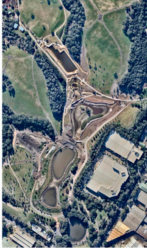
During Construction June 2014
