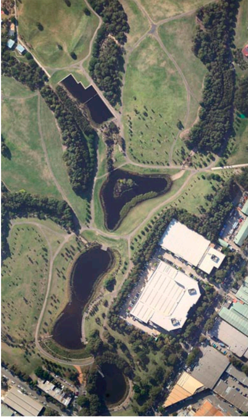
Before Construction April 2013
