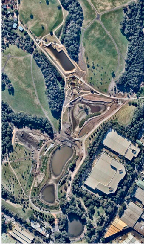
During Construction June 2014
