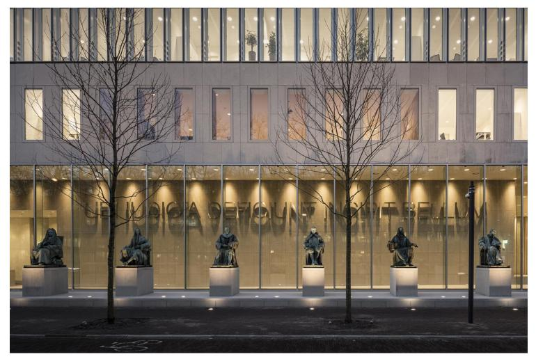
The windows on the floors above are of unified glazing, in panels of 90 cm with 10-cm joints, stretching the full height of the upper façade. There is an even division of vertical planes over the whole façade and the slender columns per window disappear in the radical rhythms of the frontage. From outside, the façade seems to have no supporting columns. The entire concept is grounded in a single design detail.
