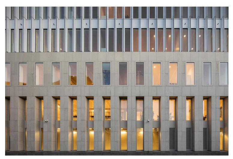
All workspaces have lofty ceiling heights of at least three meters. Usually in office Buildings, spent air is pumped away through air pipes that take up a lot of room in ceilings. In the Supreme Court building, the jambs of the door frames evacuate this air from the rooms into the open areas and ventilators above transport the spent air out. A labyrinthine construction in the frames prevents sound leakage between workrooms and hallways.
